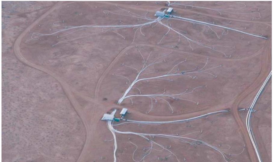
Figure 4. Wellfield at Beverley (undisturbed desert at far left).
